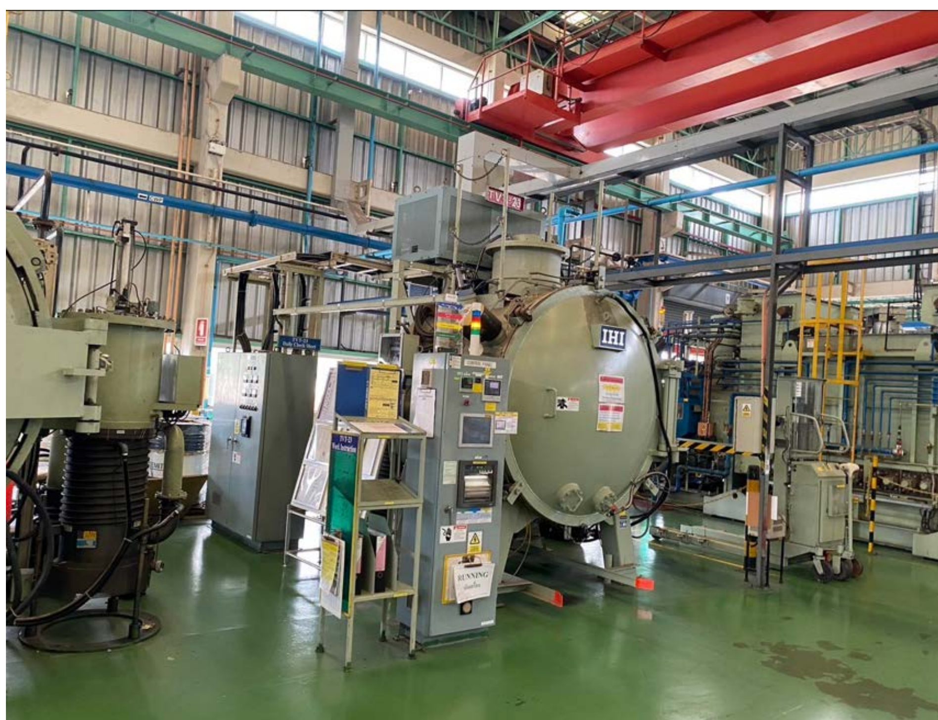
Industrial Heat Treating Furnace with CQI-9 requirement
