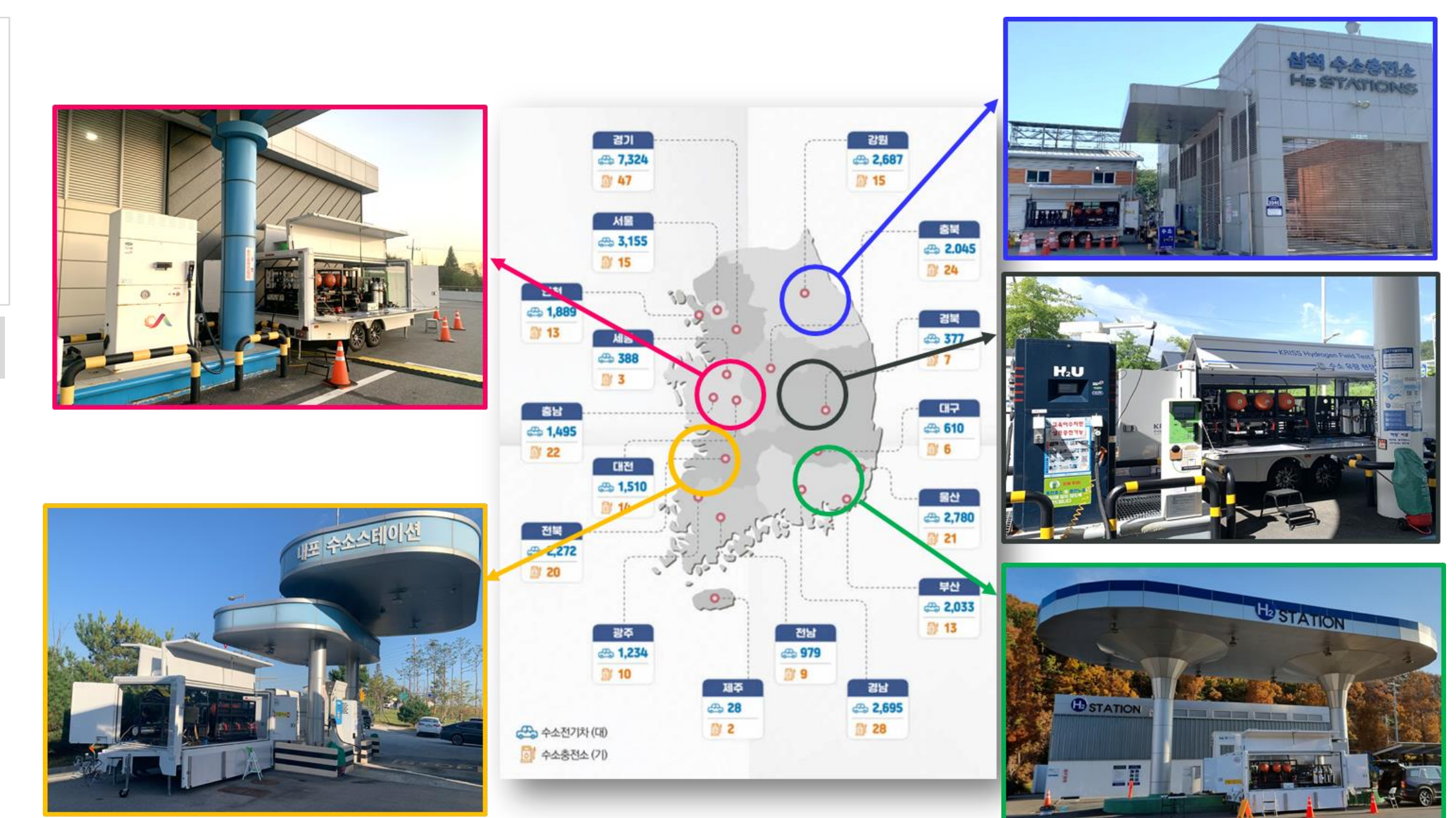
On-site test of KRISS HTFS at the Hydrogen station in Korea from 2022-2025
