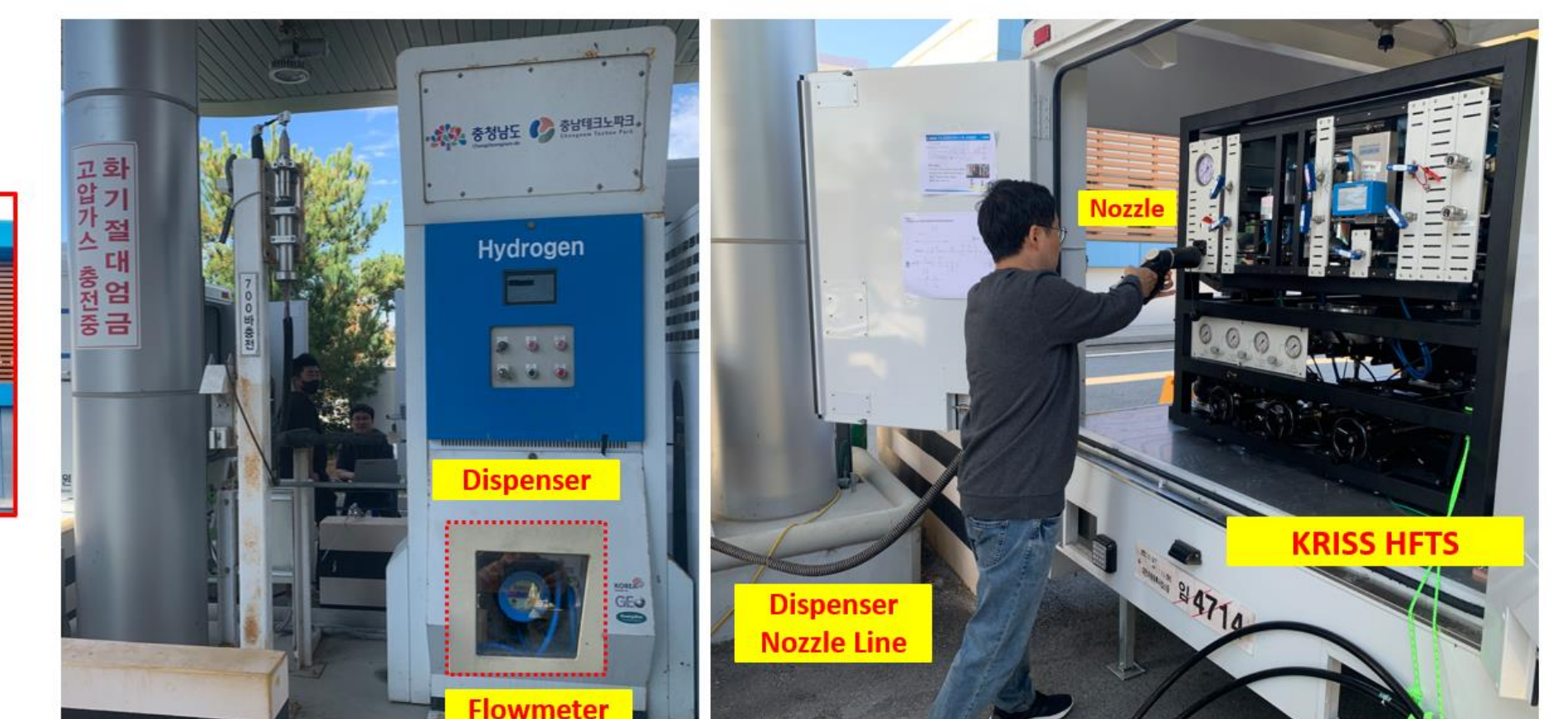
Connecting nozzle of hydrogen dispenser to KRISS HTFS
